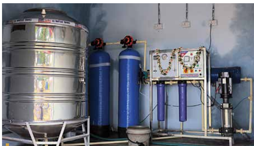
Built a water purification plant at Toopranpet
